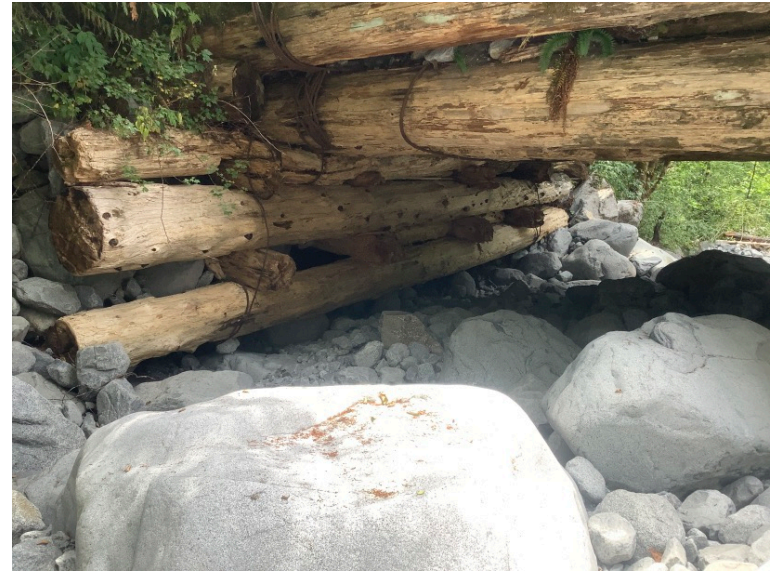
Left Bank Abutment when facing downstream
