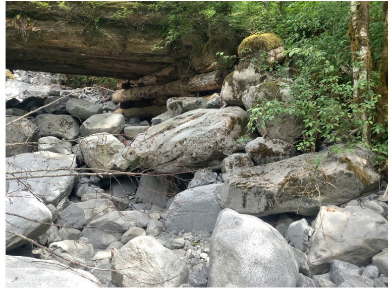
Left Bank Abutment when facing downstream
