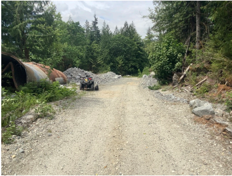
Bridge deck, viewing to right approach
