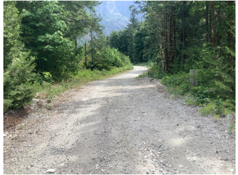
Bridge deck, viewing to left approach
