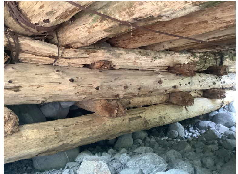
Left Bank Abutment when facing downstream
