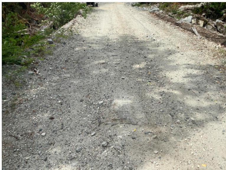
Left approach, stringer end visible
