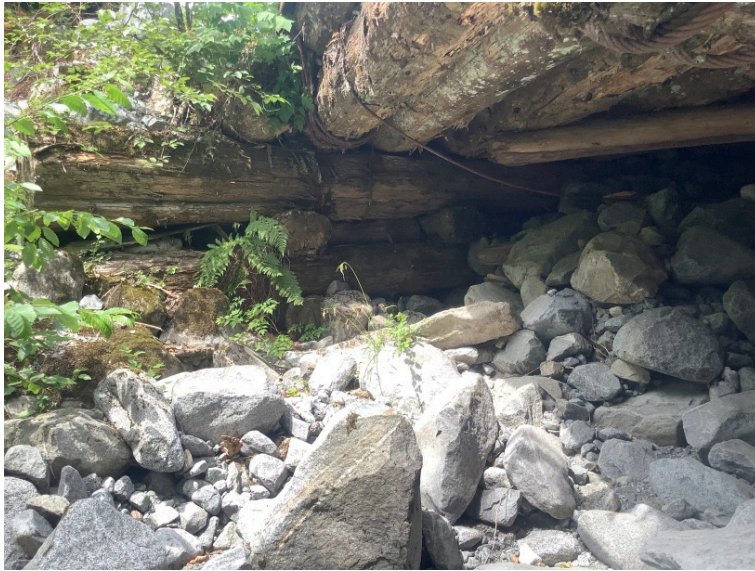
Right Bank Abutment when facing downstream
